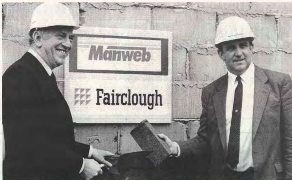
David Elderton, right, hands a brick to the Chairman, Bryan Weston, for him to cement into place
