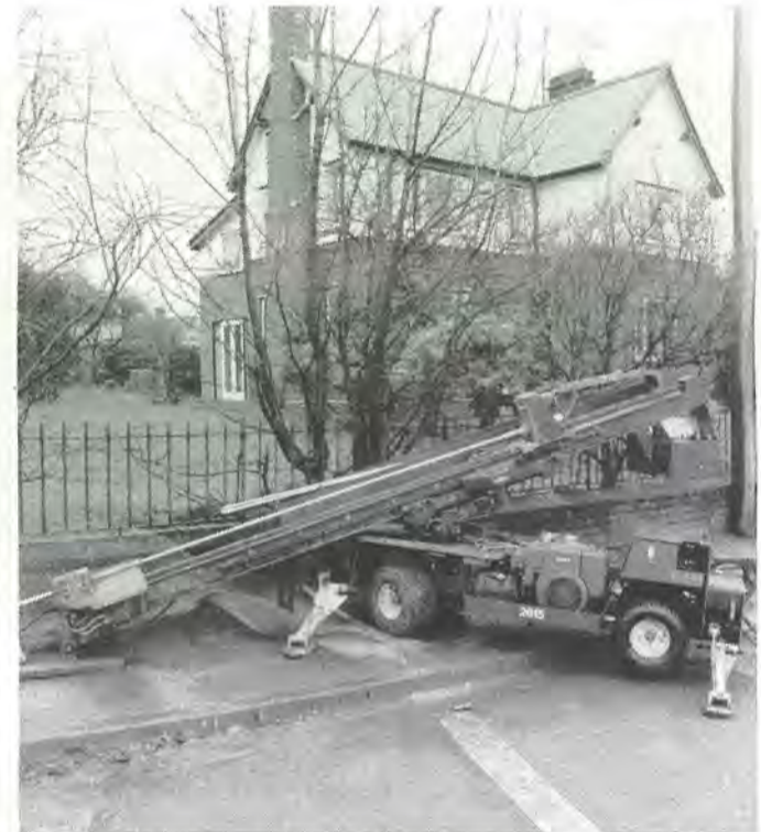
Above: Preparing to send the tunnelling-head underground. Below: The micro-tunnelling-jet goes under the road, whilst the heavy traffic thunders by uninterrupted
