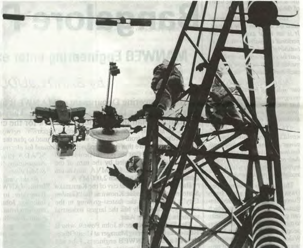
The fibre-cable-wrapping machine starts out from a tower
