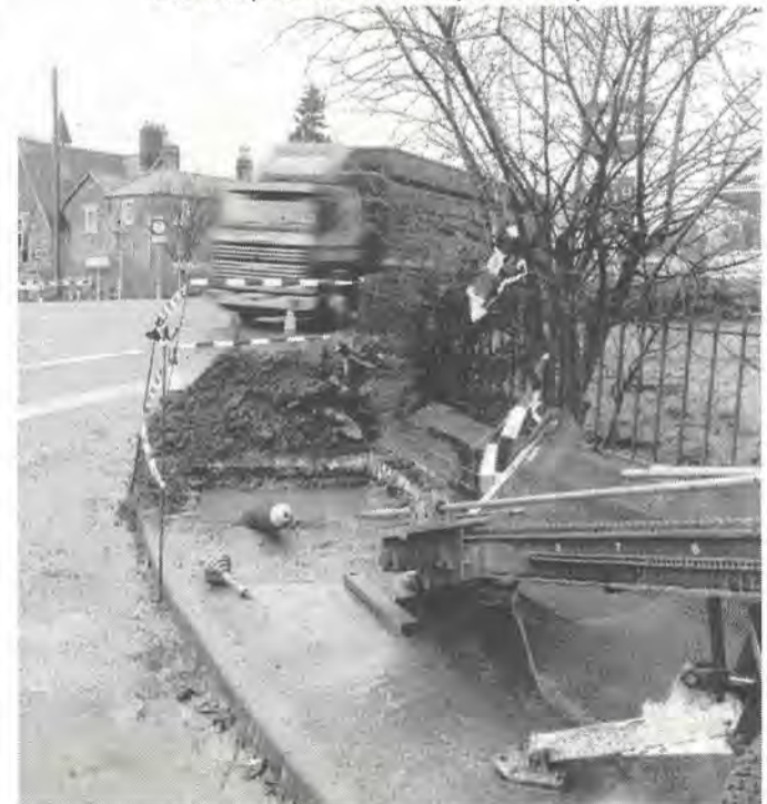
Above: Preparing to send the tunnelling-head underground. Below: The micro-tunnelling-jet goes under the road, whilst the heavy traffic thunders by uninterrupted
